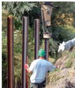
Battage des supports
