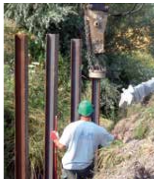
Battage des supports
