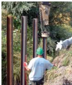
Battage des supports
